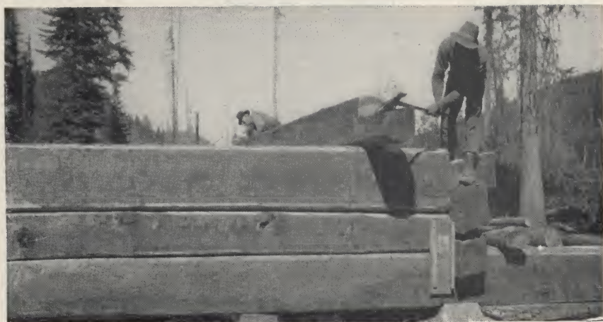
FIGURE 29.—Framing hewed timbers.
