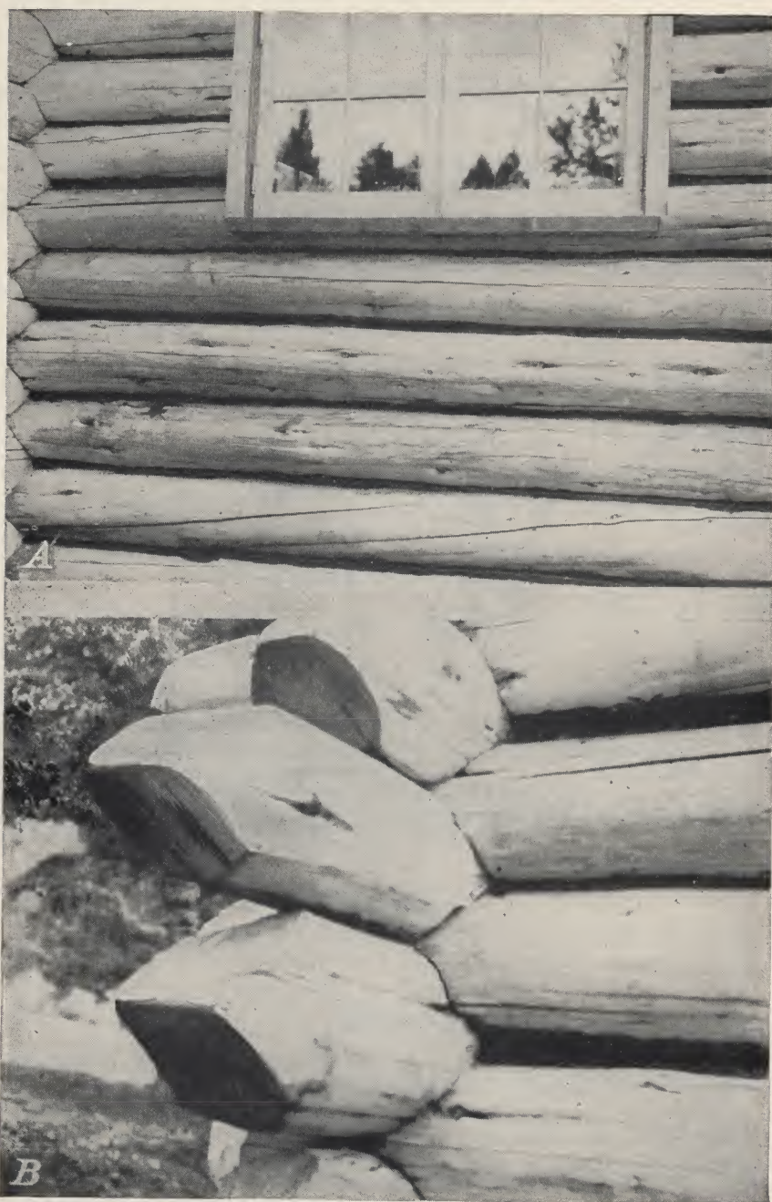
FIGURE 24.—Examples of tight joints well calked. A, Interior calking; B, exterior calking.
