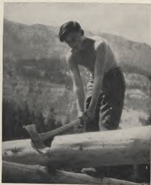
FIGURE 5.—Chopping the notch in a saddle corner.
