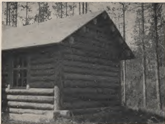
UPRIGHT OR GROOVE AND TENON CORNER
