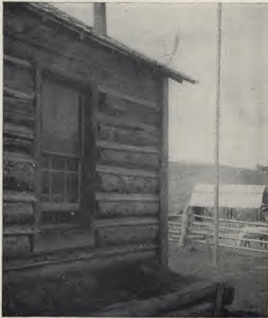
FIGURE 26.—Wood daubing strips.
