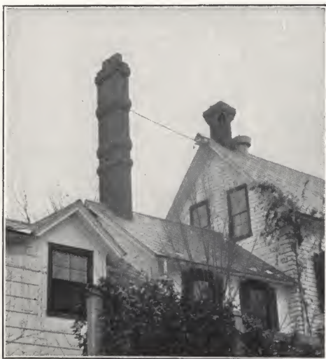
FIGURE 6.—Several extensions were necessary before this chimney would draw properly on account of the wind deflected from the nearby wall.
