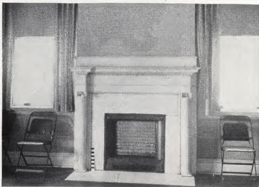
FIGURE 33.—In regions where natural gas is plentiful and in cities, fireplaces of this type, burning gas with a flickering flame, are frequently used as an auxiliary to the main heating plant. Some types have imitation logs of metal perforated for gas jets.
