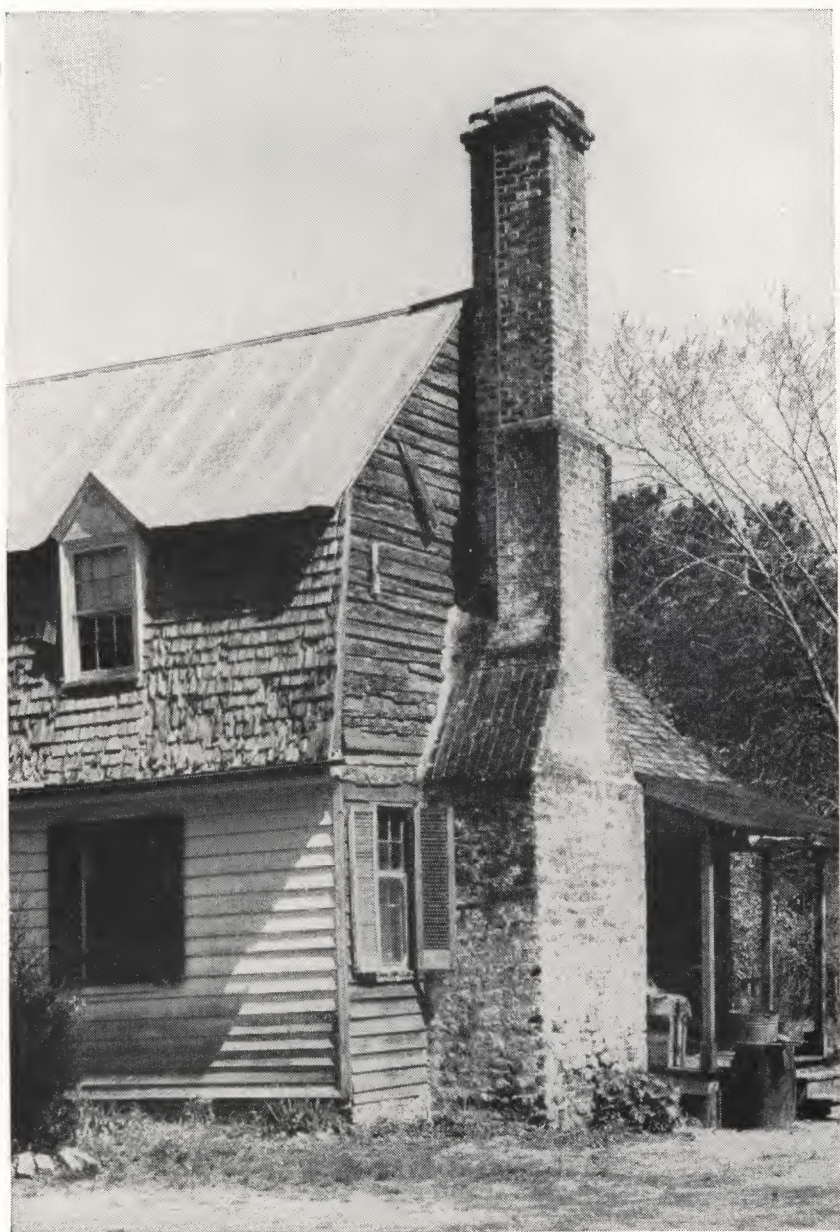
FIGURE 10.—This Williamsburg chimney shows the pains taken to make the chimney attractive. The three flues are arranged as a T with well-bonded withes between them. Often four flues were used in the form of a cross.
