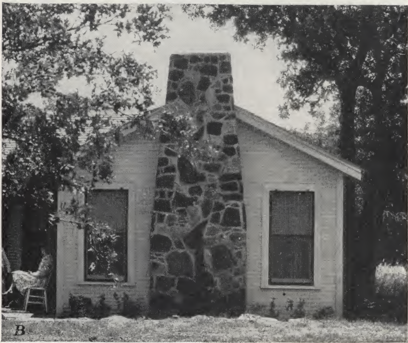
FIGURE 5.—Two pleasingly designed fireplace chimneys that fit into their surroundings. A , This chimney stands in the clear and should provide a good draft; B , a chimney under overhanging trees is likely to backdraft. Contrast the appearance of these two chimneys with that of figure 3.
