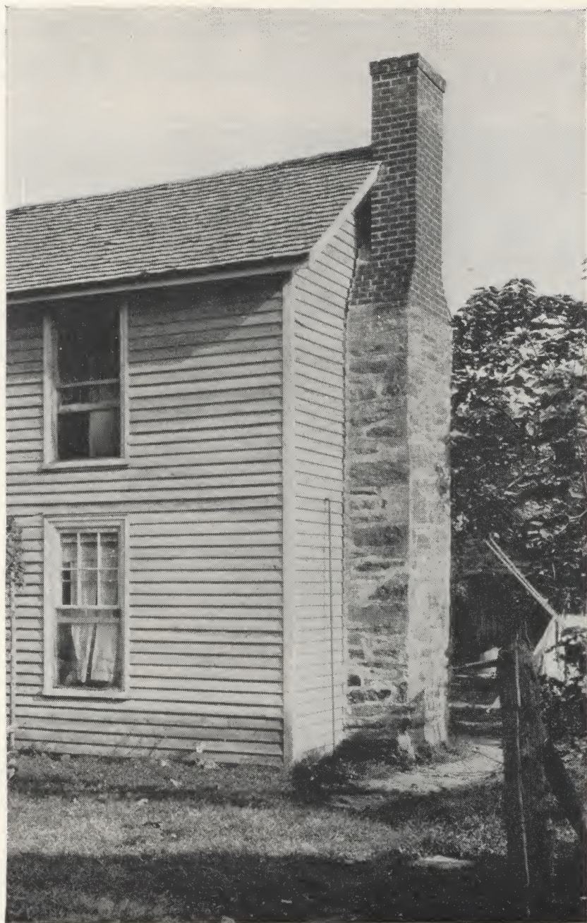
FIGURE 2.—Heavy masonry chimneys of this type are still being built in rural areas. The thick walls, with unlined flues, are in good condition after 75 years of continuous use.
