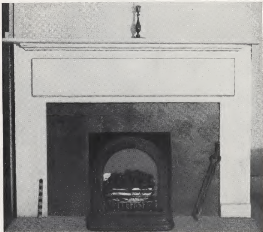
FIGURE 26.—Fireplaces originally intended for wood were frequently bricked up, and small cast-iron units of this type were built in, since the large openings required for wood were wasteful when coal was used. This was a very popular type of grate for hotel and private bedrooms about 1860 and can still be seen in old houses in coal regions. Note the plain and neat mantel of wide plank.
