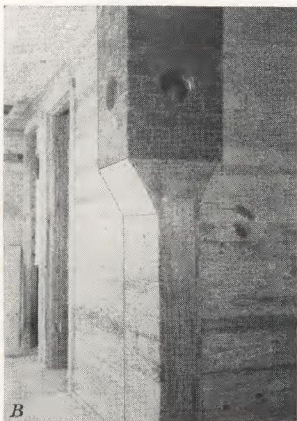
FIGURE 7.— A , A good foundation extending below the soil affected by frost. This chimney is well protected from ground moisture by the concrete carried above the surface; B , an insecure foundation. Supporting a chimney in this manner is a dangerous practice.
